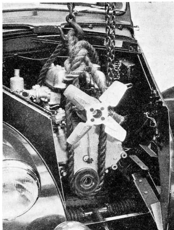
Fig. AA.24. Lifting the engine from the frame.
