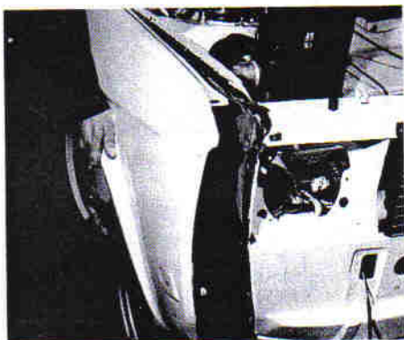
10.7 Lifting the wing from a 45 model
